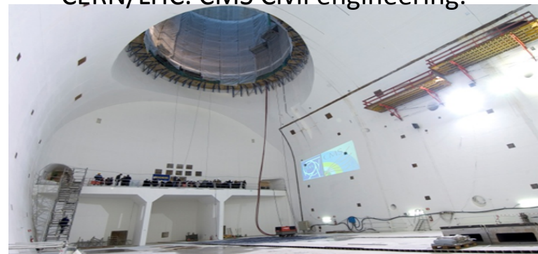
CERN/LHC. CMS Civil engineering.
