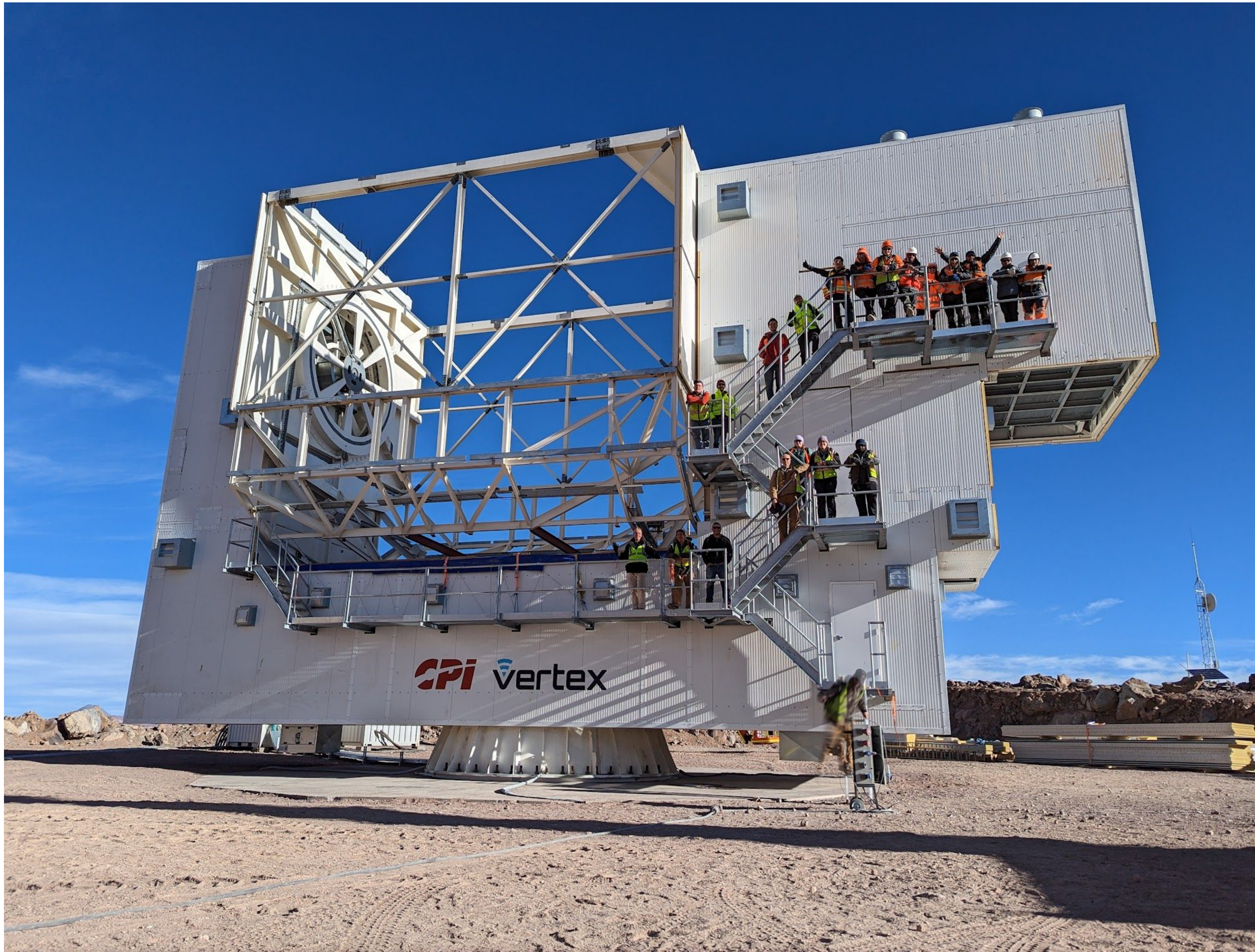
Simons Observatory Large Aperture Telescope mechanical structure on site, 2023
